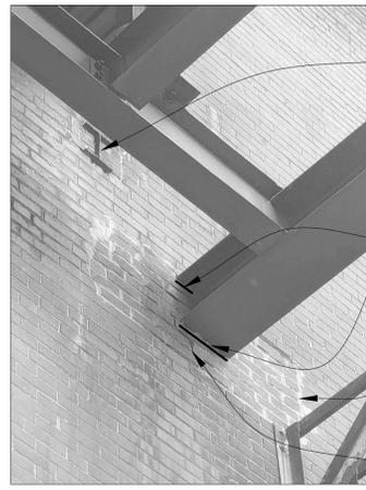
INSTALL NEW PRE-FINISHED METAL FLASHING W/ TOOLED SEALANT - SEE E4/A501
