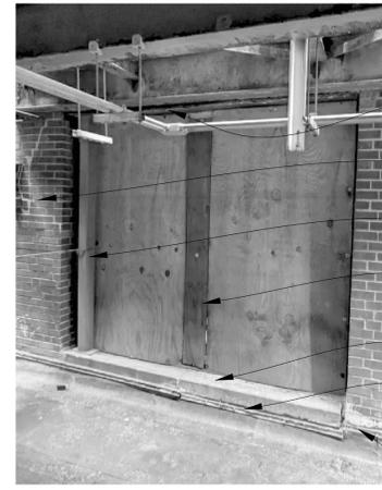
EXISTING CORRODED STEEL PLATE LINTEL TO REMAIN
