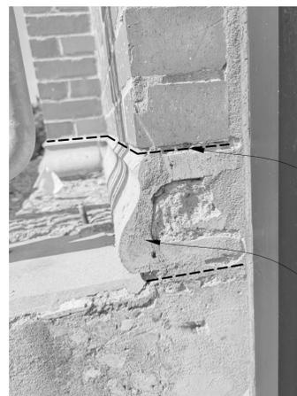
SEE C4/A501 FOR TYPICAL DIMENSIONS AT THIS PROFILE. REPLACE ONLY WHERE INDICATED - PATCH W/ REPAIR MORTAR AT ALL DAMAGE AT OTHER LOCATIONS. CLEAN & COAT TERRA COTTA AFTER OTHER REPAIRS ARE COMPLETE
