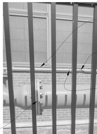
REMOVE EXISTING SEALANT AND BACKING MATERIAL @ PERIMETER OF OPENING (TYP.); INSTALL NEW SEALANT WITH BACKER ROD/BOND BREAKER
