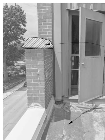
REMOVE EXISTING STONE COPING @ ASSOCIATED FLASHING(S); INSTALL NEW TREATED WOOD BLOCKING, FLASHING(S), & PRE-MANUFACTURED METAL COPING - A1/A201
