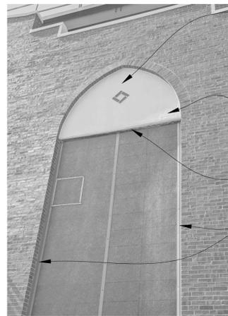
REPAIR PLASTER WHERE NOTED; FOLLOWING REPAIR - CLEAN, PRIME, & PAINT ENTIRE PLASTER SURFACE. TEMPORARILY MASK EXISTING EXPOSED BRICK TO PREVENT STAINING BY PLASTER/PAINT.
