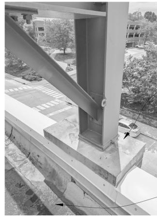
REMOVE EXISTING METAL PILASTER/PIER CAP FOR MASONRY REPAIRS. REPLACE THIS CAP FLASHING AS NOTED IN DETAILS:
