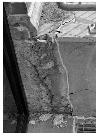
CHIP OUT AND REMOVE LOOSE CONCRETE TO SOLID MATERIAL. USE CONCRETE REPAIR MORTAR TO PATCH DAMAGED CONCRETE
