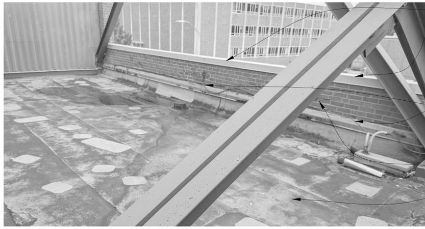
TEMPORARILY REMOVE EXISTING COPING & BLOCKING TO MINIMUM EXTENT POSSIBLE - FOR INSTALLATION OF NEW CONTROL JOINT AND OR REPLACEMENT OF BRICK AT BACK OF PARAPET; REINSTALL EXISTING COPING & BLOCKING W/ NEW SEALANT @ SAME LOCATION.
