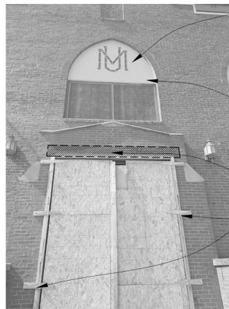
REPAIR PLASTER WHERE NOTED: FOLLOWING REPAIR - CLEAN, PRIME, & PAINT ENTIRE PLASTER SURFACE. TEMPORARILY MASK EXISTING EXPOSED BRICK TO PREVENT STAINING BY PLASTER/PAINT.
