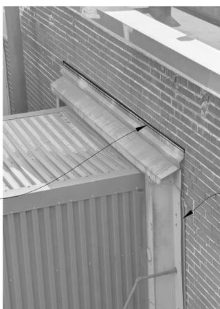
REMOVE EXISTING SEALANT AND BACKING MATERIAL @ SIDES OF OPENING (TYP.); INSTALL NEW SEALANT WITH BACKER ROD/BOND BREAKER
