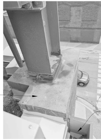
TEMPORARILY REMOVE CONDUCTOR HEAD, DOWNSPOUT, STRAP HANGERS; SALVAGE, STORE & REINSTALL AT SAME LOCATION AT END OF PROJECT
