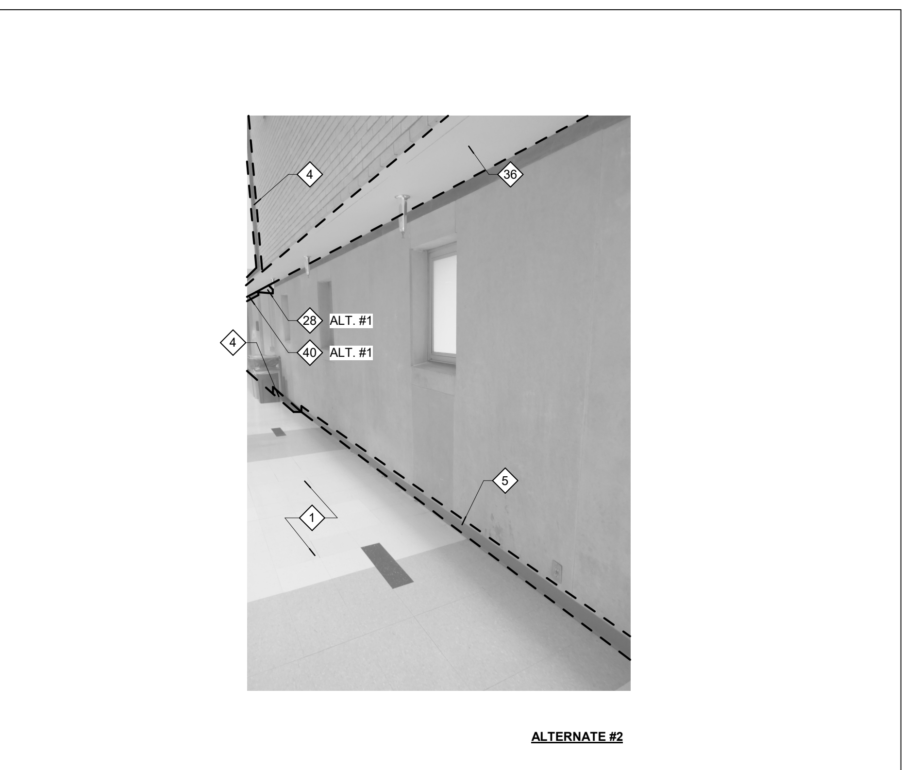
AC100B CORRIDOR - DEMO PHOTO 2 | B7
