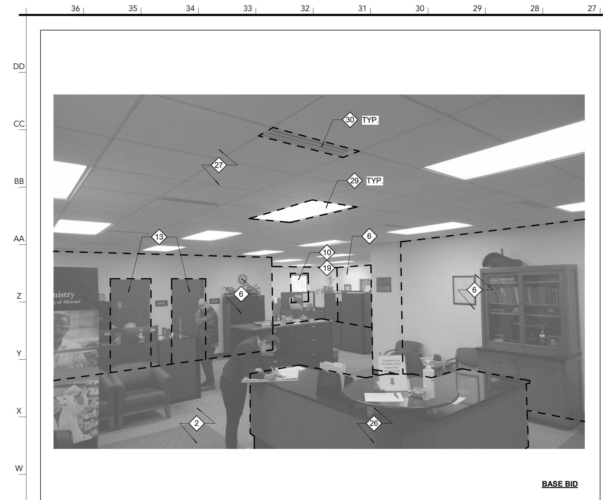
125 OFFICE - DEMO PHOTO 1 | W27
