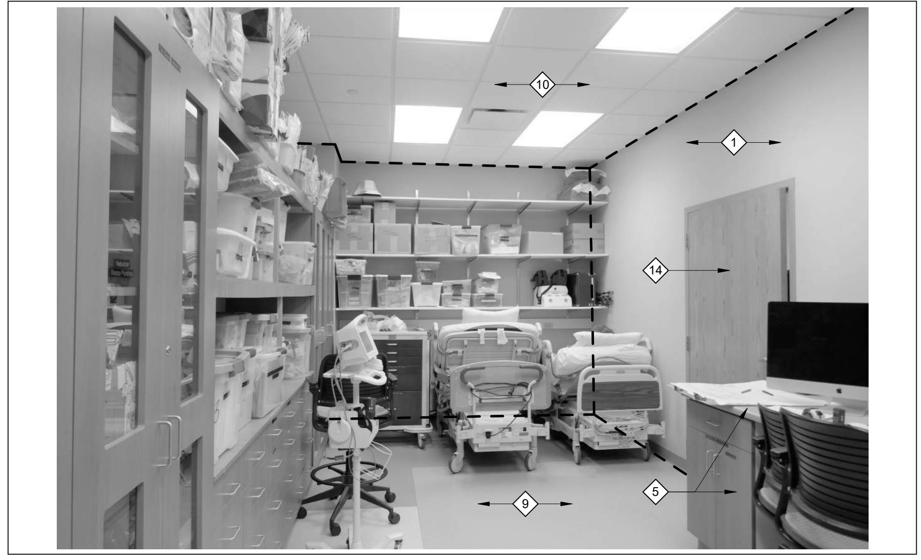
CE630A EAST ROOM PHOTO | B27
