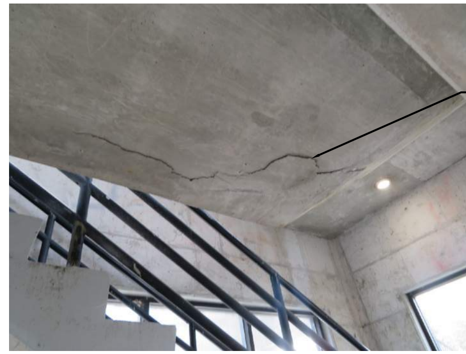
11 DELAMINATED SOFFIT AT 3RD LEVEL SW STAIR N.T.S.
