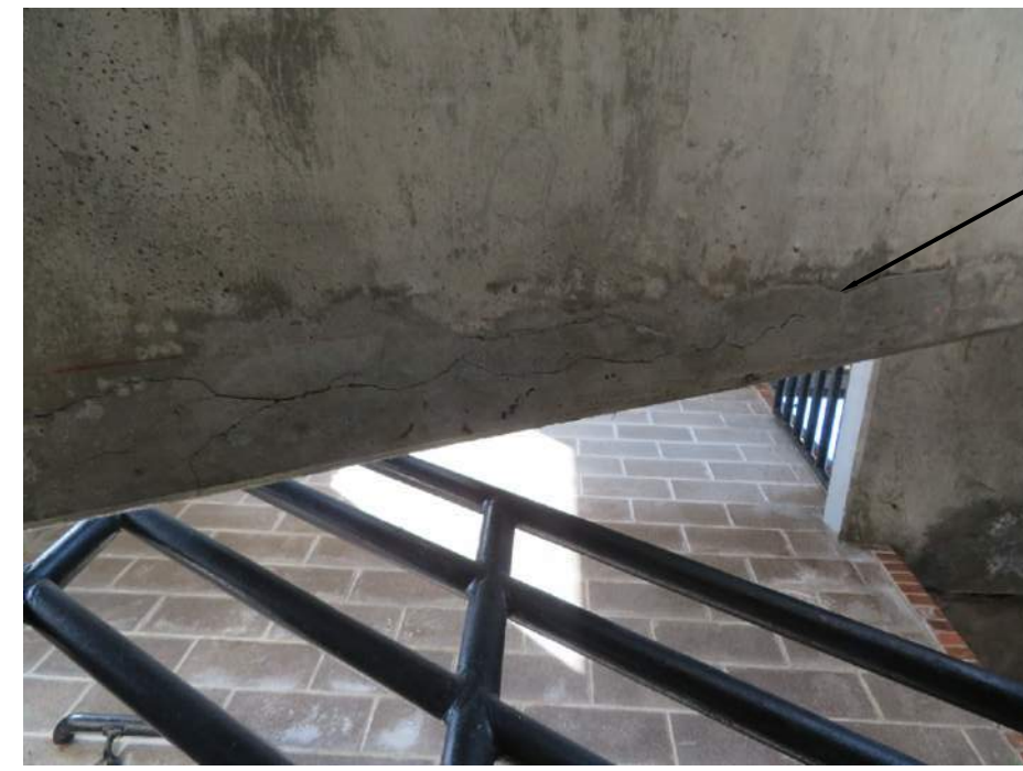
11 DELAMINATED SOFFIT AT 2ND LEVEL SE STAIR N.T.S.
