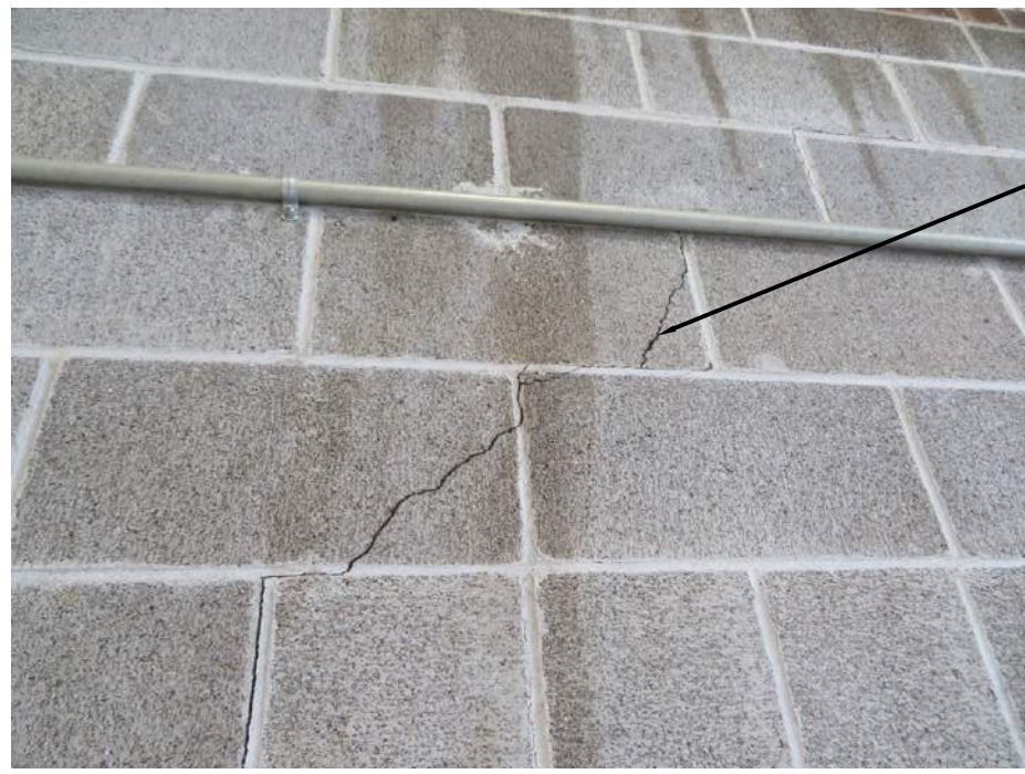
15 CMU WALL CRACK AT 3RD LEVEL SW STAIR N.T.S.
