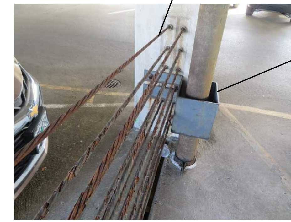
2 BARRIER CABLES AT COLUMN N.T.S.
