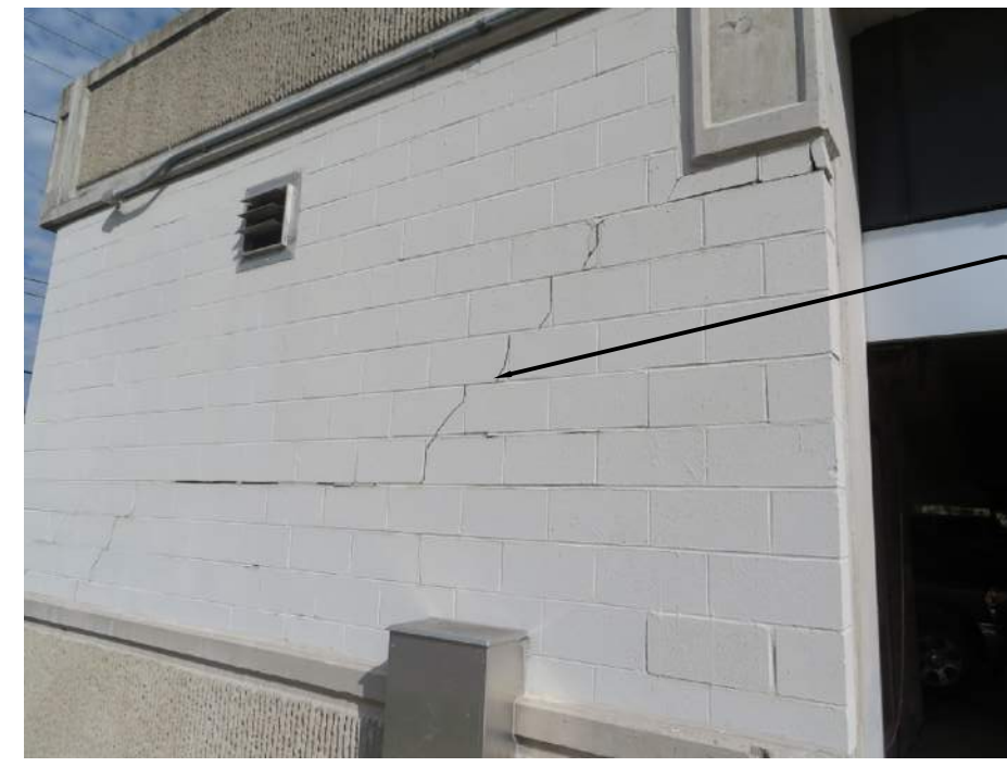
16 CMU WALL CRACK AT GROUND LEVEL NW CORNER N.T.S.
