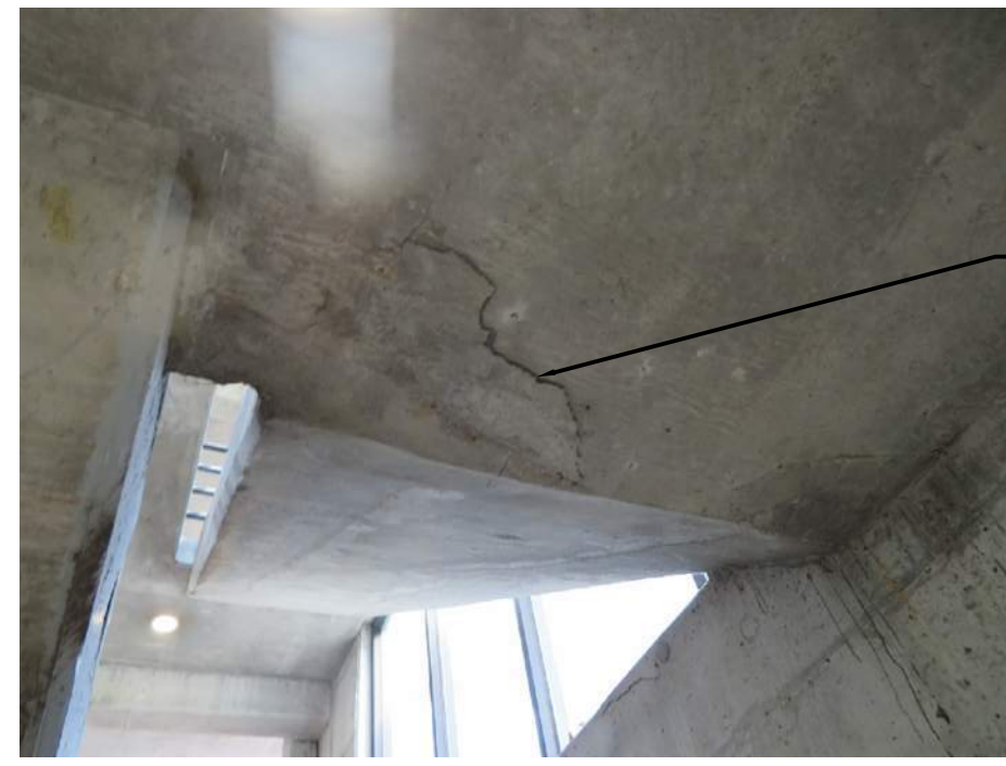
12 DELAMINATED SOFFIT AT 2ND LEVEL SW STAIR N.T.S.
