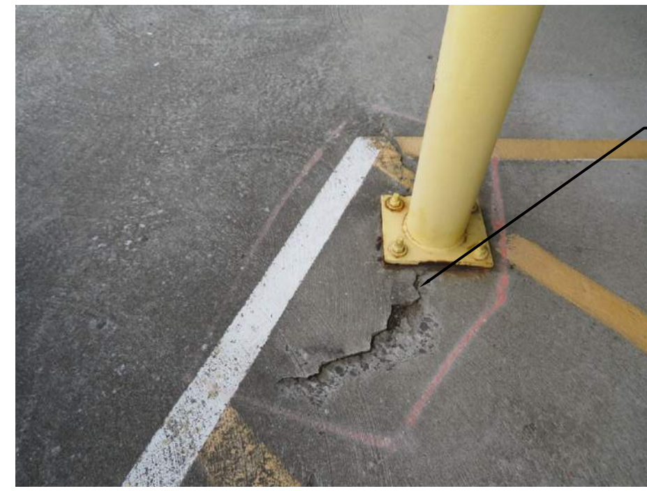
15 DELAMINATED SLAB AT 3RD FLOOR NW CORNER N.T.S.
