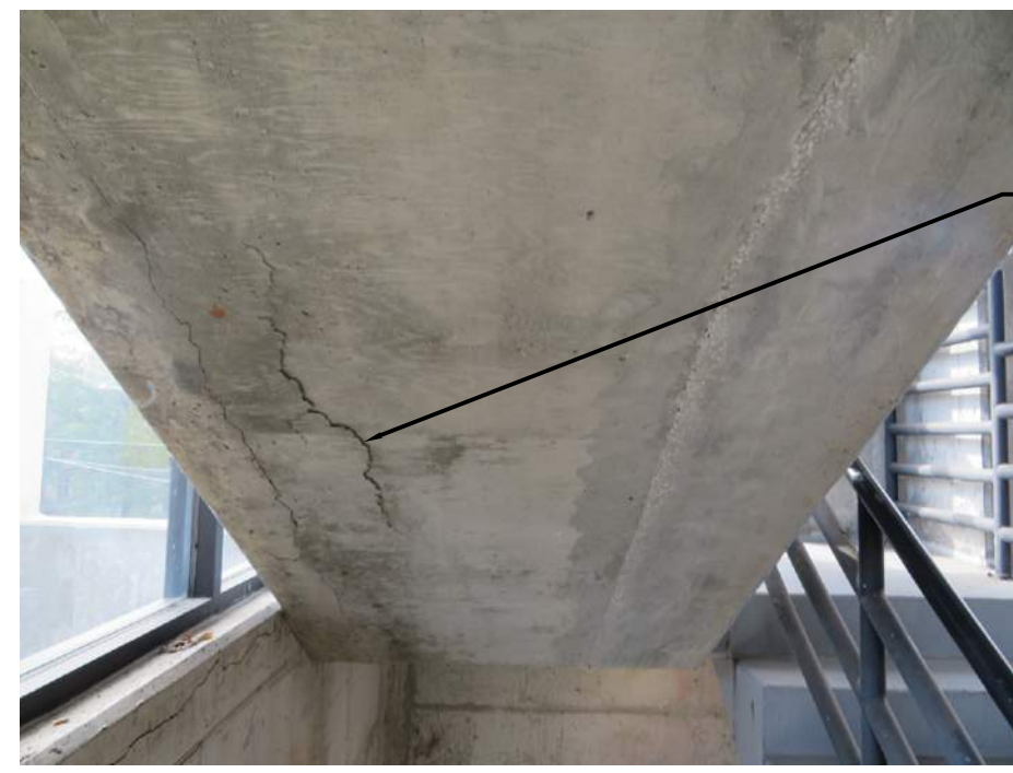
10 DELAMINATED SOFFIT AT 3RD LEVEL SW STAIR N.T.S.
