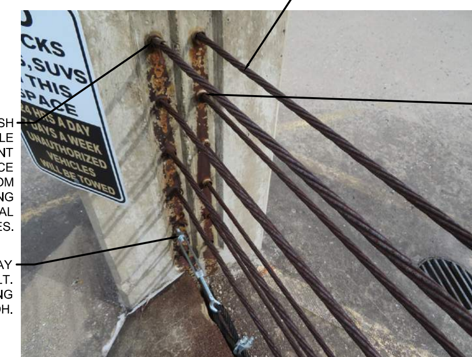
1 BARRIER CABLES INTO COLUMN N.T.S.
