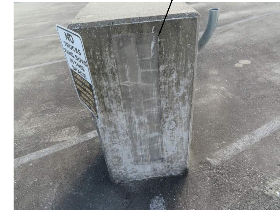
3 BARRIER CABLE GROUT POCKETS N.T.S.
