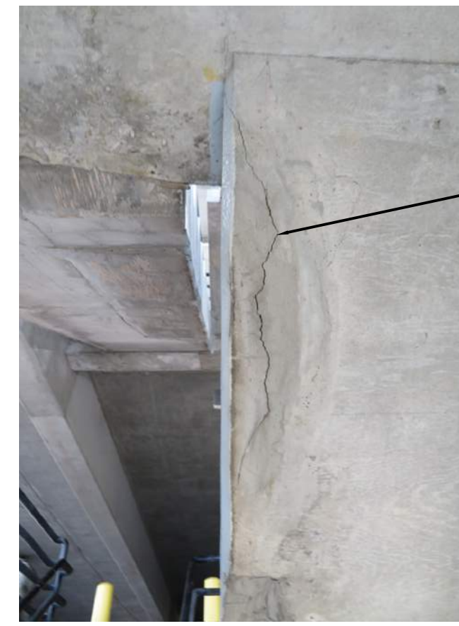
7 DELAMINATED SOFFIT AT 2ND LEVEL NW STAIR N.T.S.
