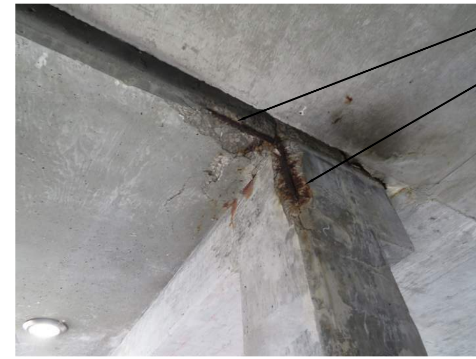
7 DELAMINATED COLUMN AND SOFFIT AT 3RD FLOOR SW STAIR N.T.S.
