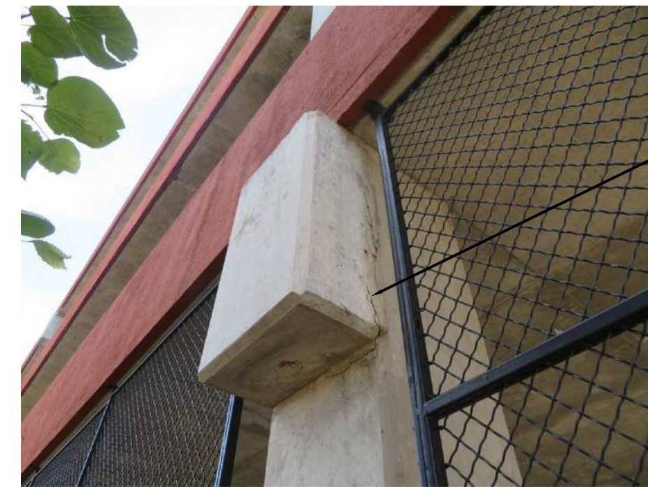
6 DELAMINATED COLUMN AT GROUND LEVEL NORTH SIDE N.T.S.
