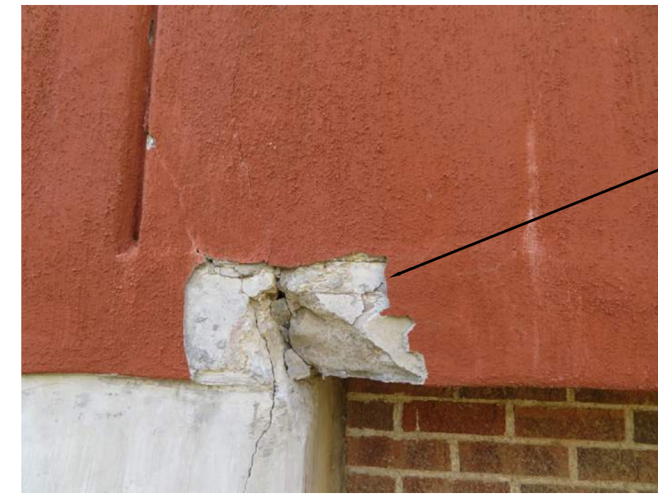
8 DELAMINATED BEAM AT GROUND LEVEL EAST SIDE N.T.S.
