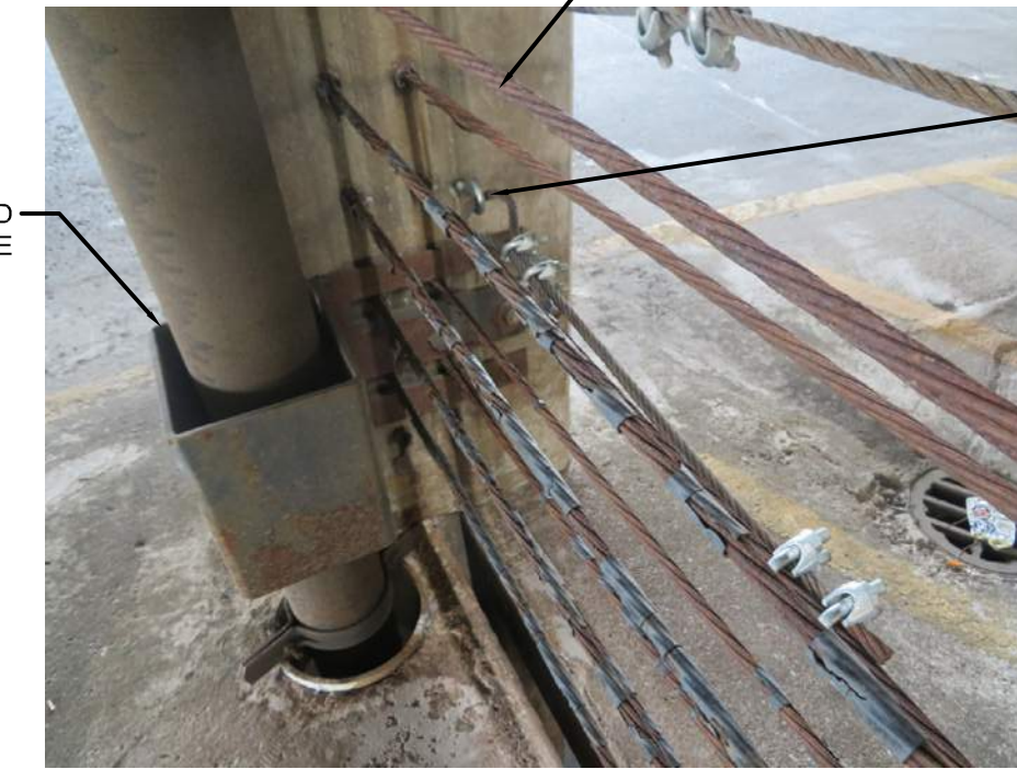
2 BARRIER CABLES INTO COLUMN N.T.S.
