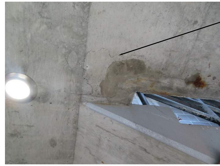
12 DELAMINATED SOFFIT AT 2ND LEVEL SW STAIR N.T.S.
