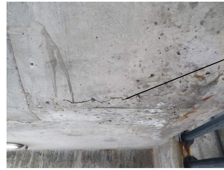
8 DELAMINATED SOFFIT AT 2ND LEVEL NW STAIR N.T.S.
