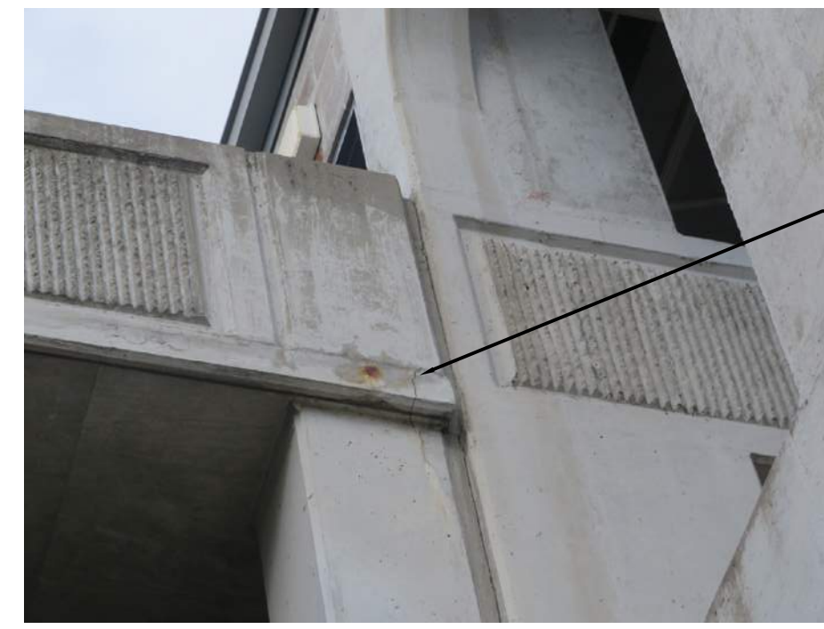
6 DELAMINATED SPANDEL AT ROOF LEVEL SE CORNER N.T.S.
