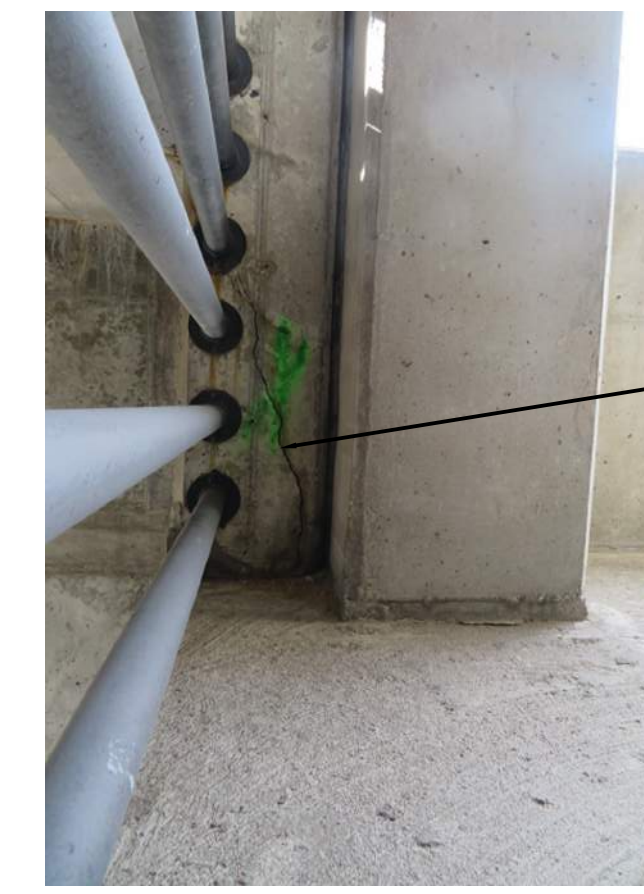
4 DELAMINATED COLUMN AT 2ND LEVEL NW STAIRS N.T.S.
