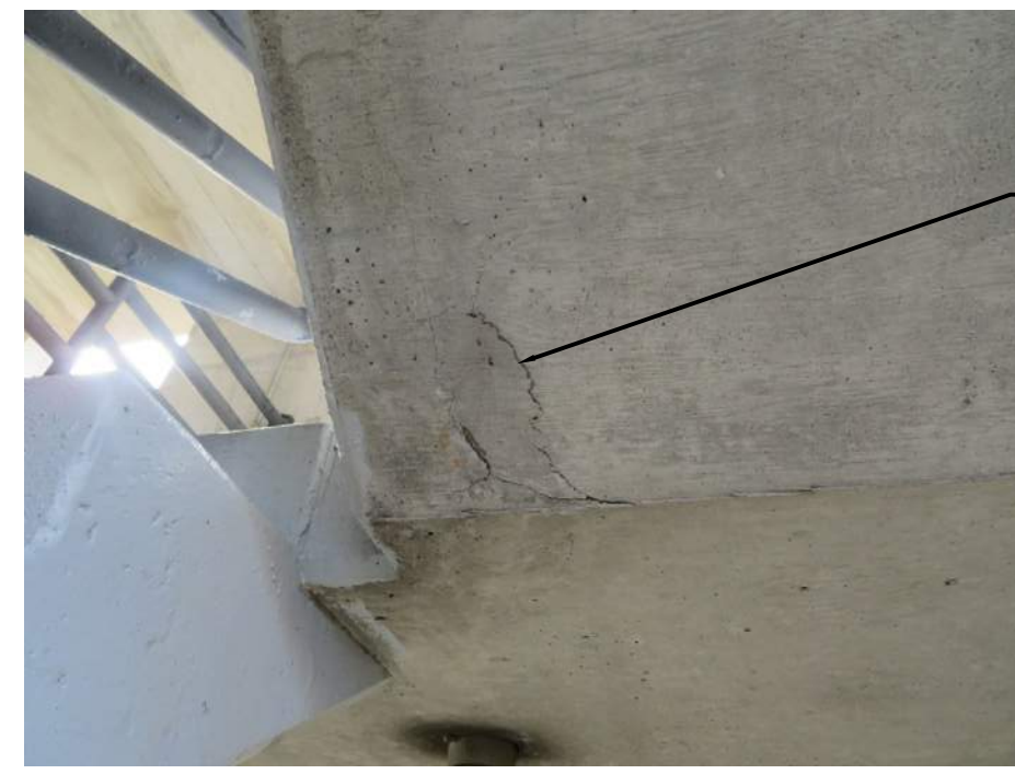
14 DELAMINATED SOFFIT AT 3RD LEVEL NW STAIR N.T.S.
