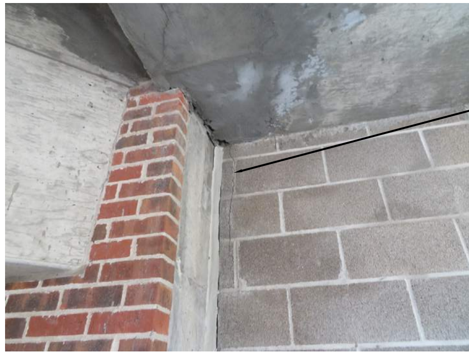
16 CMU WALL CRACK AT 2ND LEVEL SE STAIR N.T.S.
