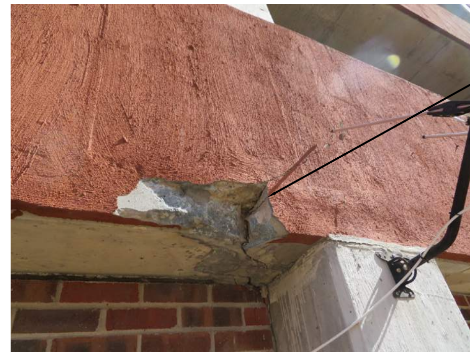
10 DELAMINATED BEAM AT GROUND LEVEL WEST SIDE N.T.S.
