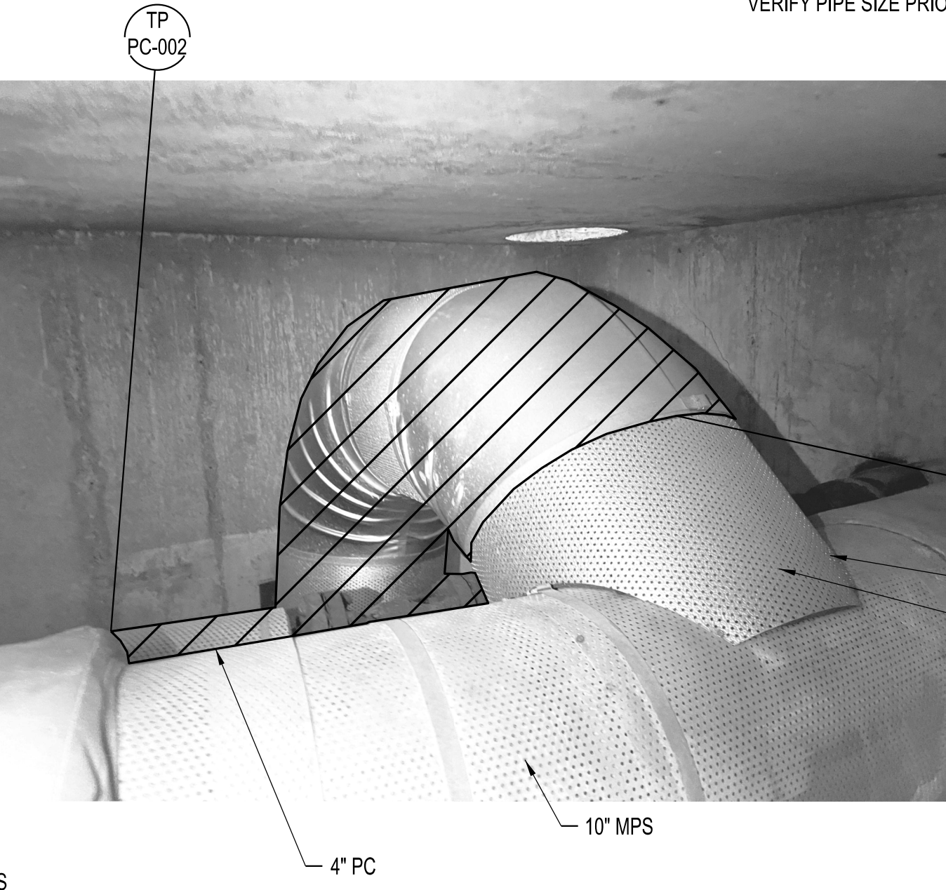
4 MPS AND PC IN SMH-421 (LOOKING NORTH) DM011
