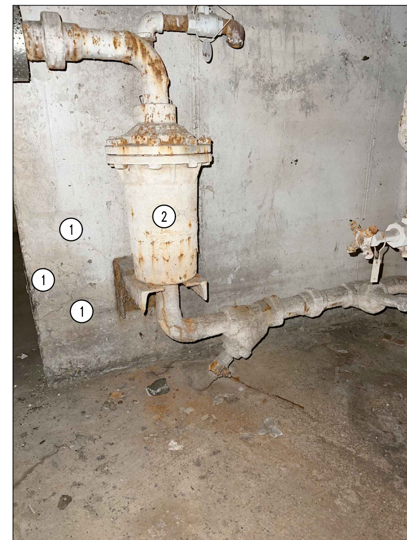
1 CONCRETE CRACKING, SEE REPAIR NOTE 4. 2 OWNER TO REMOVE PRIOR TO REPAIRS.
