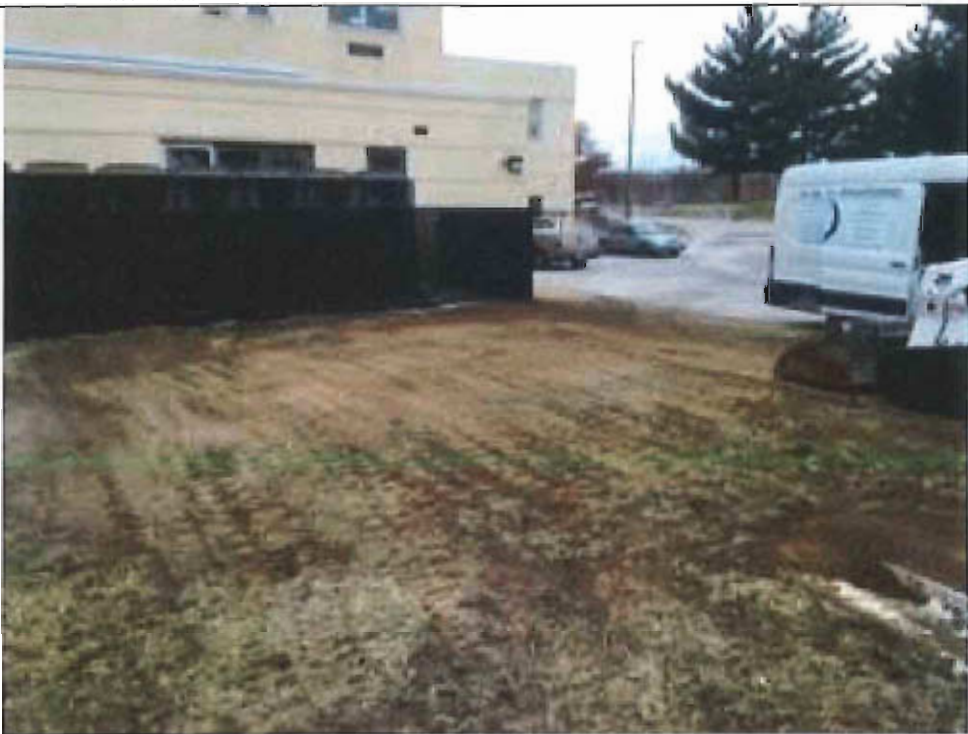
14. View of site after closure
