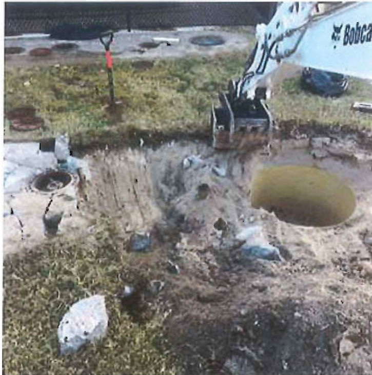
1. Removal of concrete around UST manways
