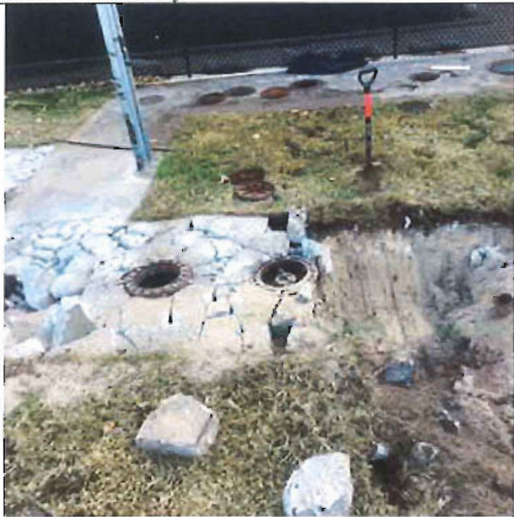
2. Removal of concrete around UST manways
