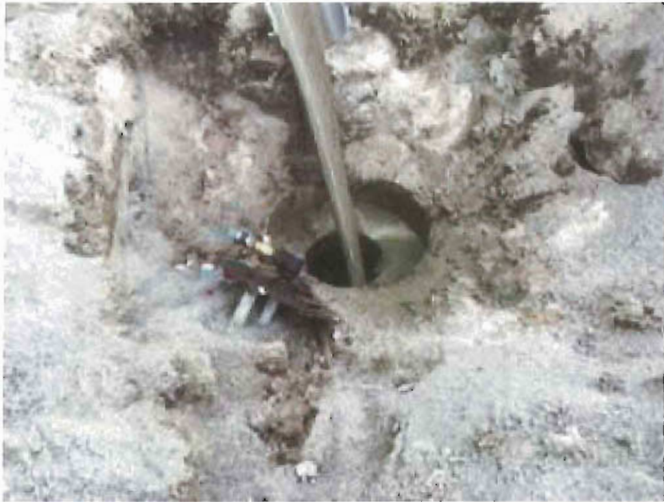
9. Concrete being placed in UST
