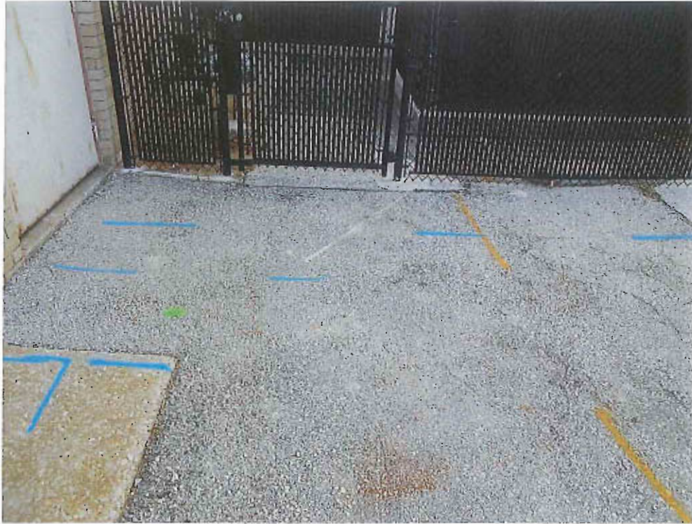
33. Utility lines in pipe trench
