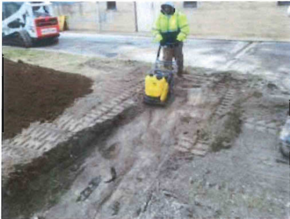
13. Compaction of fill material
