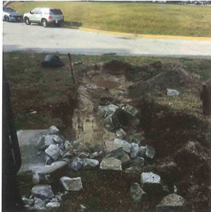
3. Removal of concrete and soil around UST manways
