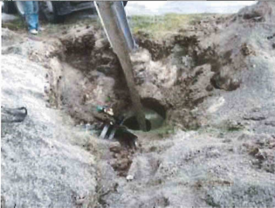
10. Concrete being placed in UST
