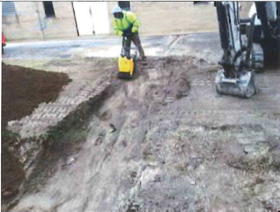
12. Compaction of fill material
