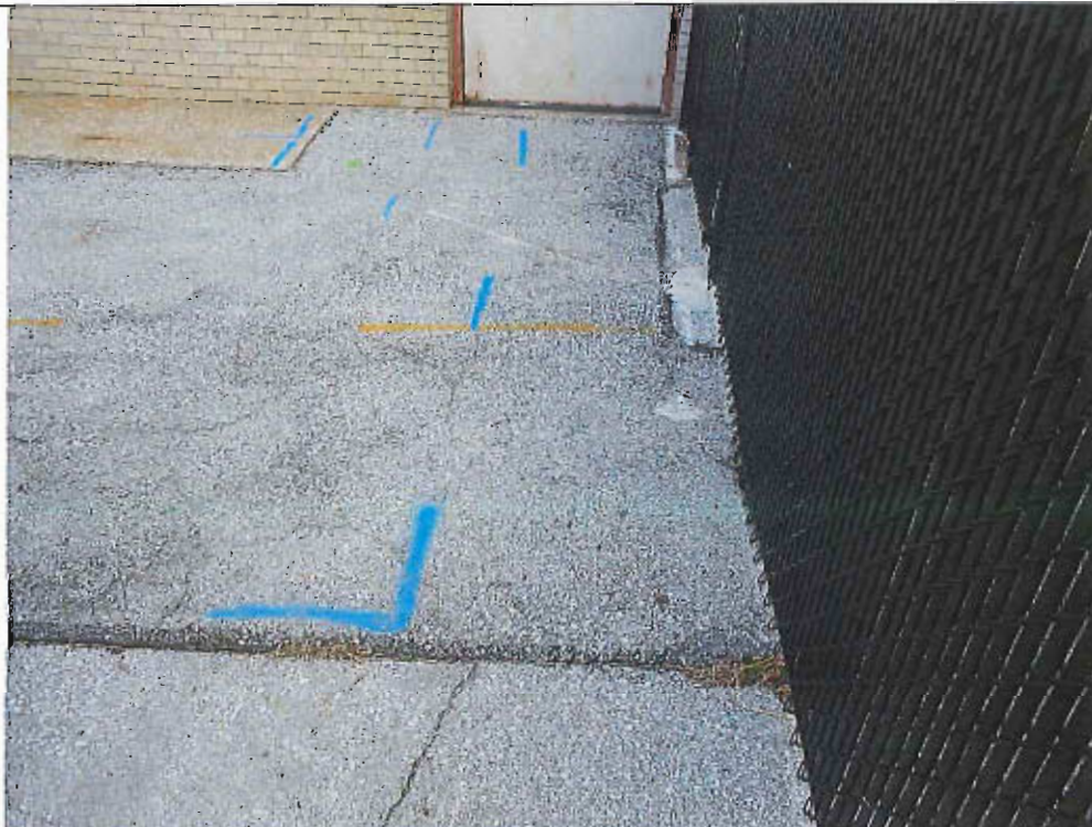
32. Utility lines in pipe trench
