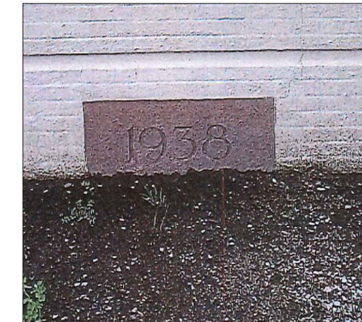
ITEM 27: BUILDING CORNERSTONE
