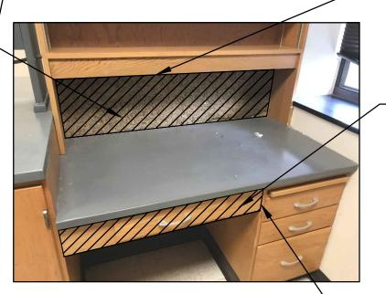
PATCH &/OR REPAIR BASE CABINETS ETR AND FILLER PANEL (ALL SIDES) AS NEEDED
