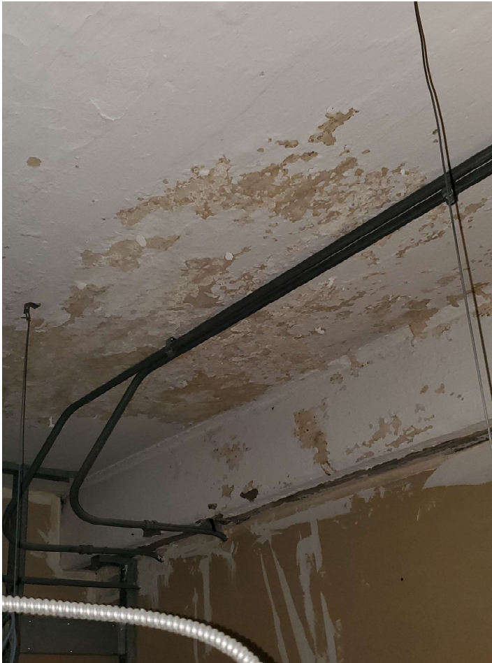
Deteriorating lead-based paint on the concrete deck
