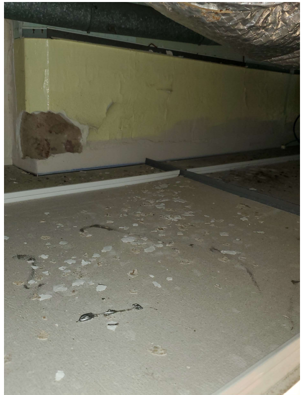
Lead-based paint debris on ceiling tiles
