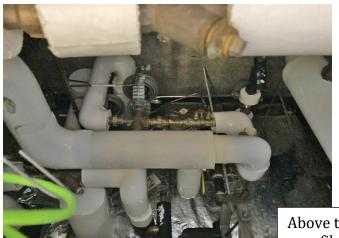
Above the drop ceiling of 3E-11, new fiberglass pipe insulation, duct insulation, bare concrete deck above
